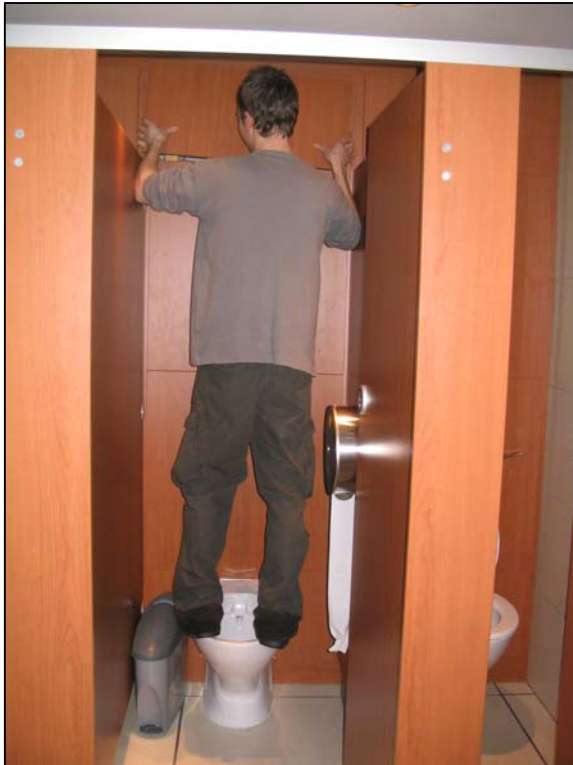
Figure 5.3 Removing panels to fit Save-a-flush bags
