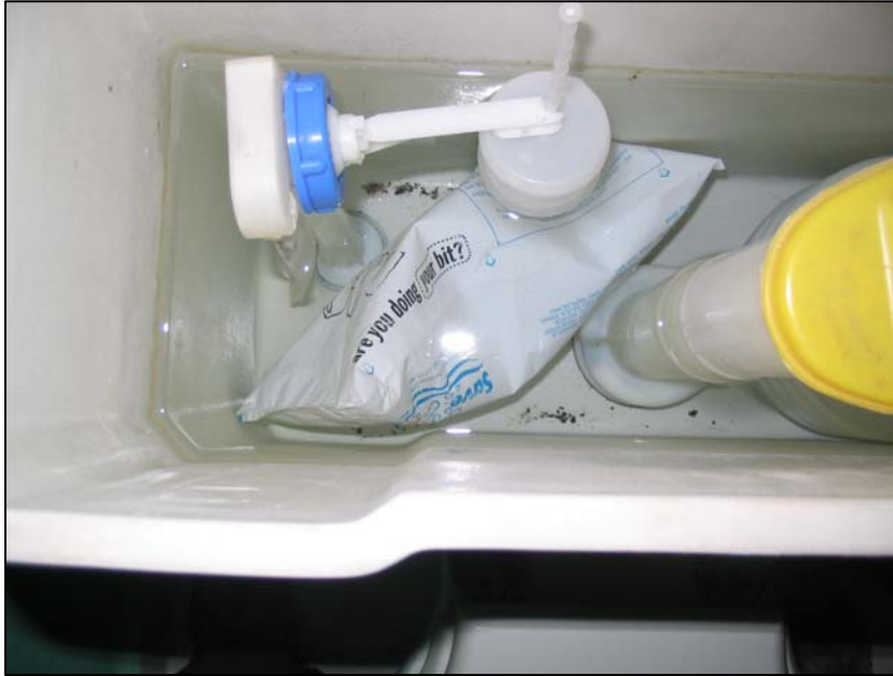
Figure 5.1 Save-a-flush bag in cistern
